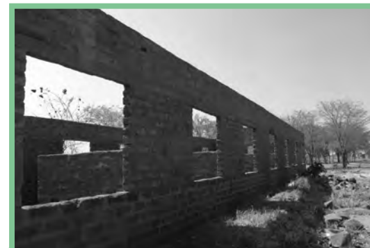
MWA-funded dormitory in progress
